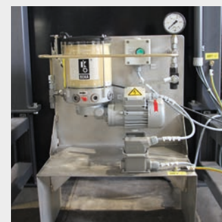
Central lubrication system equipped with progressive distribution
